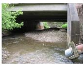
Sediment deposition has reduced flow capacity under several bridges significantly. This can create a pinch point during high flow events.
