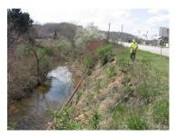
MP3 along McKnight Road has several pipes that are at severe risk of collapse as the streambank has eroded away, leaving them suspended and without support.
