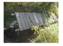
Improperly and illegally constructed bridges and streamside structures can wash away and block streams, increasing flood damage.
