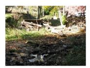
A deteriorated railroad tie retaining wall is no longer serving its original purpose and could contribute flooding debris to create dams in a storm event.
