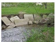
Efforts to armor stream bank with concrete slab are not completely effective.
