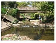
Even the most sturdy bank armoring designs have proven unequal to the force of West little Pine in its southern reaches. Here, a road is in jeopardy if the wall fails.
