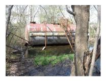
An inactive storage tank near the stream presents a significant hazard of stream contamination or damage to vegetation or structures if dislodged and floated downstream.
