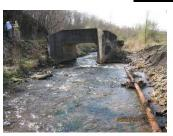
Pipes that were formerly buried within the streambank have become exposed pipe along lower reaches of Willow Run due to erosion. If carrying sewage, potable water or fuel, this pipes are now vulnerable to corrosion and damage during storm events.
