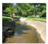
This section of West Little Pine portrays a history of homeowners struggling with increasing pressure on the streambanks behind their properties. The increased height of the retaining wall in background, and erosion at the top of the wall in the foreground show the need for reduced flows and better streambank management.
