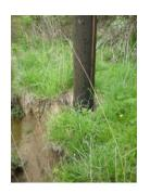
Some of the erosion has put utilities at risk such as this electrical or telephone utility pole.
