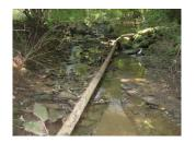
Numerous exposed pipes exist in the stream channel, including some that are totally corroded.
