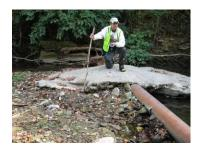
Erosion also threatens utility infrastructure. Here a pipe that had originally been cemented over is now exposed.
