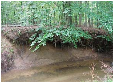
Significant Erosion due to Excess Runoff
