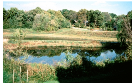
Wet Pond BMP to Reduce Erosion
