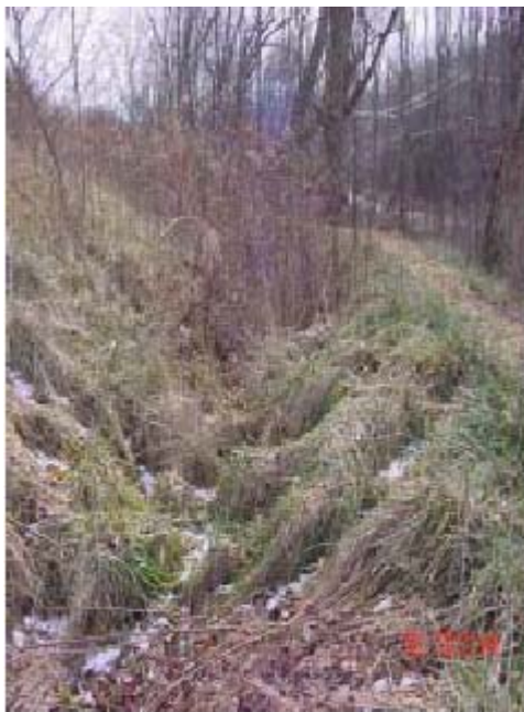
Narrow, vegetated recharge trenches follow land contours and take on a naturalized appearance.
